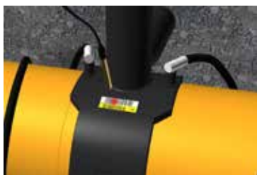
Figure C.35: Input of welding parameters
