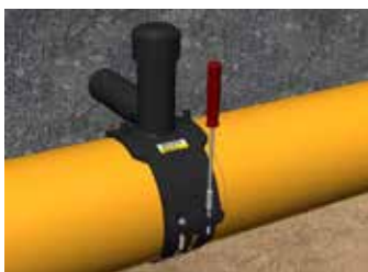
Figure C.34: Mounting the saddle
